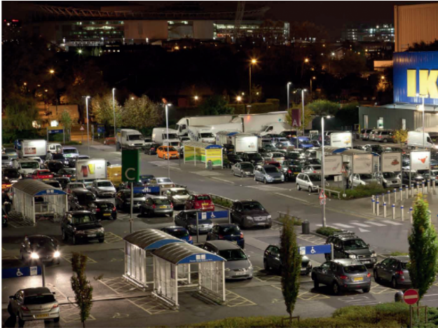
Figure 13: In the outdoor car park, 62 road luminaires installed at a height of 8 m and spaced at 8–9 m, each containing 40 LEDs consuming 94 W use microwave sensors for dimming. The average illumination in the car park is 100 lx, with a uniformity ratio of 0.57 [Reproduced from Ref. [40], with kind permission].
