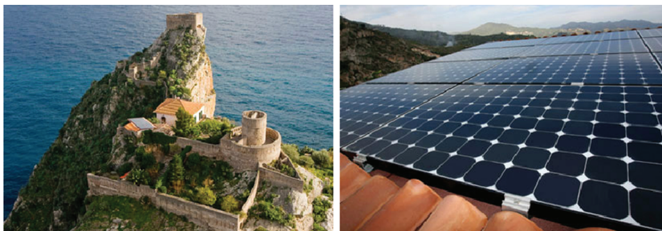
Figure 5: Installed in 2009, the BIPV array of the Sant'Alessio Castle comprises 20 black frameless modules, covering 33 square metres. [Image courtesy, SunPower Corporation.]
