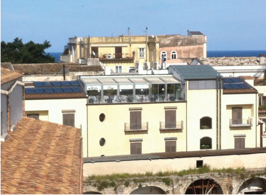
Figure 9: The BIST forced circulation system on the roof of Hotel Porta Felice in Palermo. [Photo courtesy of the authors.]
