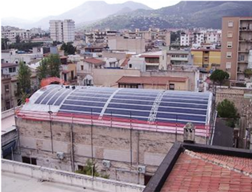
Figure 11: The flexible 20 kW PV array on the roof of the Teatro Crystal, in Palermo, uses a polyolefin membrane supporting the amorphous silicon modules. [Photo courtesy of Medielettra.]
