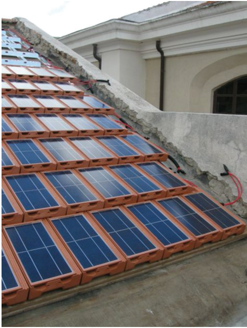
Figure 2: PV tiles over the roof of a church in Sicily’s Zafferia. The 5.5 kW PV array was realized in 2013, with the approval of the Superintendency of Arts. [Image courtesy of Wegalux.]
