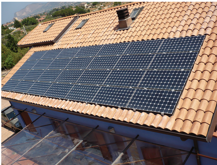
Figure 4: The BIPV roof of this home, located in Sicily's Casteldaccia, comprises of black solar modules replacing the corresponding tiles. [Image courtesy of the home's owner.]
