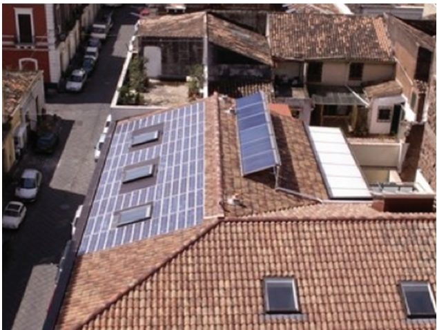
Figure 3: The PV roof of Hotel Rigel, in Catania, is comprised of polymer-supported PV modules covering 55 square metre, with an overall 6 kW power. [Image courtesy of Brianza Plastica.]
