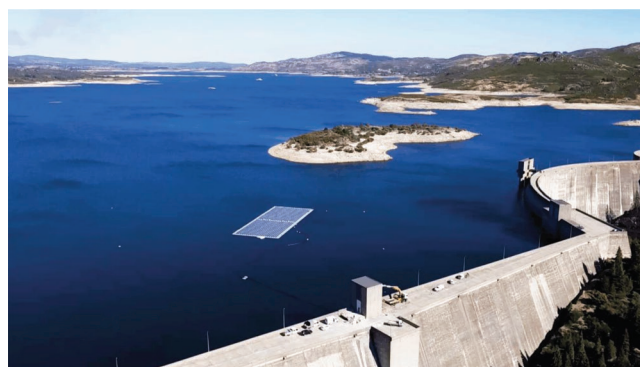
Figure 1. The 218 kW floating solar plant on Portugal's Alto Rabagao hydroelectric dam. Connected to the grid in late 2016, the floating system supports 840 PV modules, with bottom anchoring designed to meet a maximum depth of 90 m and a level variation of 30 m. Photo reproduced with permission from Ciel & Terre.
