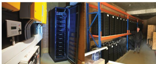
Figure 6. The 48 kWh battery system (left) and the 160 kWh saltwater battery (right) used in an off-grid avocado plantation in Pemberton, Australia. (Image courtesy of Unlimited Energy Australia).
