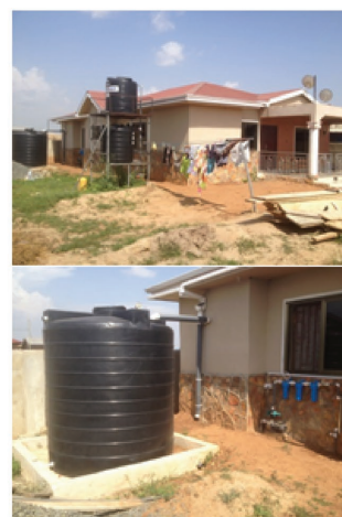
Figure 1. Domestic rainwater harvesting system providing potable water to 20 households in Ghana's Accra. 1 = gutters; 2 = downpipe; 3,4 = pipe bend; 5 = T-piece; 6 = flush diverter; 7 = tank; 8 = cast foundation; 9 = distribution and disinfection system. Reproduced with permission. [22] Copyright 2015, SINTEF.
