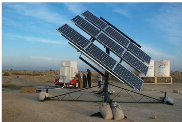
Figure 2. One of the solar-powered water purification systems installed in Iraq between 2010 and 2012 to supply 729 rural villages and small cities with clean potable water after a cholera outbreak in 2009. Reproduced with permission. [24] Copyright 2015, Solaropia.
