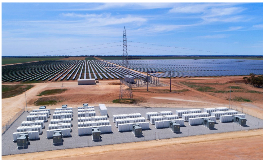
Figure 1. The 25 MW/50 MWh energy storage system next to the Gannawarra Solar Farm, Australia. Reproduced with permission. [5] Copyright 2019, Edify Energy.
