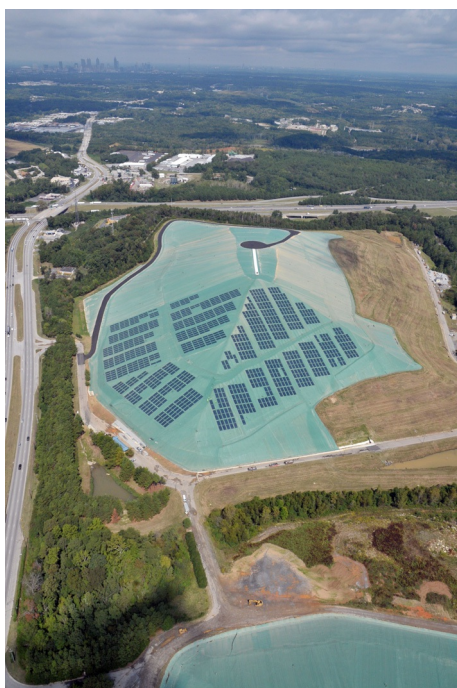
Figure 4. Hickory Ridge landfill near Atlanta, hosting a 1 MW PV with solar-exposed geomembrane on the southwest and southeast slopes of the landfill. Image reproduced from Wikipedia, with kind permission.
