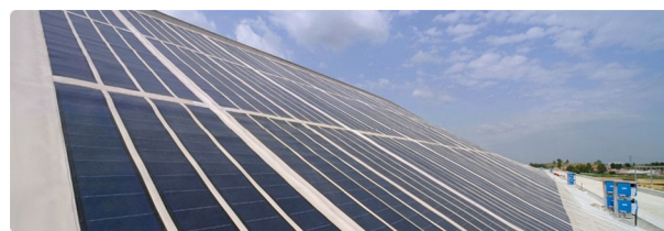
Figure 2. Part of the 752 kW PV flexible array at Rome’s Malagrotta landfill. Reproduced from Ref. [13], with kind permission.
