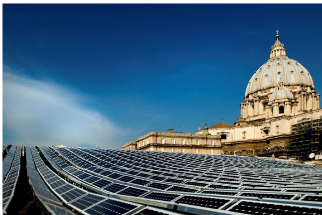
Figure 1. Section of the 225 kW PV plant on the roof of Paul VI Hall, next to St. Peter's Dome: 2394 tailor-made solar modules perfectly follow the sweeping, wave-shaped roof in concrete.
