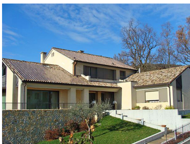
Figure 5. Home in Italy rooftop with solar bent tiles. The elegance and all functional properties of the earthenware rooftop are retained, but the roof now generates clean electricity every day. [Photo courtesy of Industrie Cotto Possagno].
