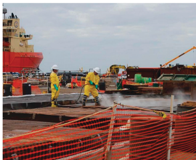
Fig. 5 Workers in Louisiana using limonene-based cleaning agent PES-51 to decontaminate equipment used to clean large vessels following the Macondo well blowout and Deepwater Horizon explosion on April 20, 2011. [Image reproduced from ref. 20, with kind permission.]
