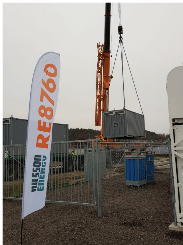
Figure 4. Funded by the European Union within the project hydrogen mobility europe (H2ME) and cofunded by fuel cells and hydrogen joint undertaking (FCH JU), the hydrogen refueling station in Mariestad, Sweden, generates H 2 from water using electricity from the PV park adjacent to it. On November 2018 the first containerized electrolyzer was delivered to the hydrogen filling station. Reproduced with permission. [62] Copyright 2018, Nilsson Energy.
