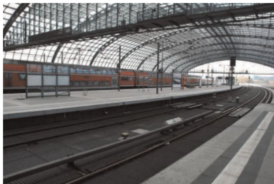
Figure 16. Glass-glass photovoltaics on the Lehrter train station in Berlin. (Photo credit: jameswagner.com).
