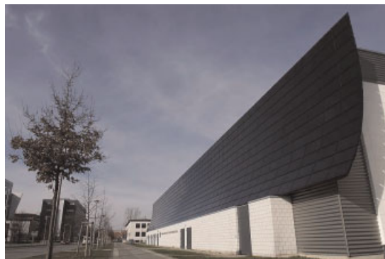
Figure 14. The elegantly shaped solar wall at Ferdinand-Braun Institute in Berlin costed 250 000 € for 39 kWp. (Photo credit: Sulfurcell).
