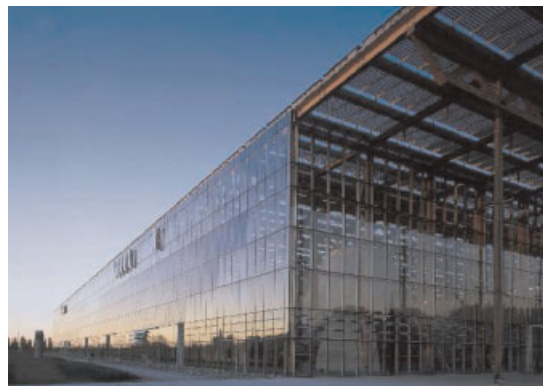
Figure 17. Academy and building multi-use Mont-Cenis, Herne, Germany. This building contains an academy, hotel, offices and library, all wrapped in glass of 180 m of length, 72 m of width and 16 m of height. (Photo credit: Bipv.ch).
