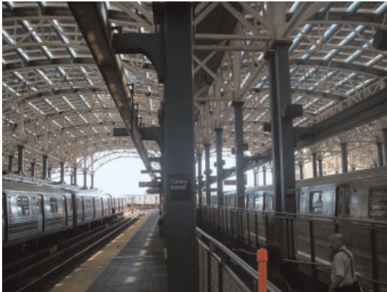
Figure 1. Rated at almost a quarter of a megawatt, the Stillwell Avenue Station in New York is among the largest PV plants in the US. (Photo credit: Klingon65 on Flickr.com).
