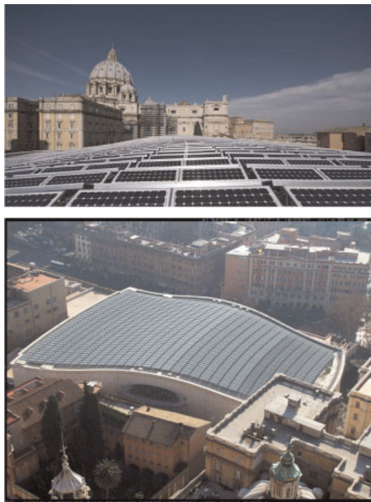
Figure 11. The BIPV plant on the roof of the Vatican 'Paolo VI' hall is magnificent example of philological restoration coupled to clean electricity generation. BIPV at its best. (Photo credit: energia e ambiente Srl).
