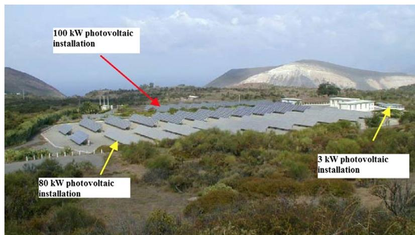
**Figure 1.** The PV plants, comprised of different silicon-based solar modules, installed in the island of Vulcano, Sicily, in 1984. After more than 30 years, the plant has recorded a modest performance deterioration [Reproduced from Ref 11, with kind permission].
