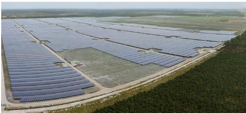
**Figure 6.** The 300 MW plant in construction in Cestas, near Bordeaux. The modules have a East-West orientation to exploit the sun radiation from early morning to late evening [Reproduced from Ref 28, with kind permission].
