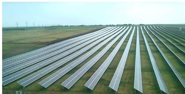
**FIGURE 1** The Yelshanskaya 25 MW photovoltaic park in the Orenburg region supplies power to the grid since 1 July 2019. Using only components made in Russia, the plant is expected to produce 30.5 million kWh annually. [Image courtesy of Hevel Energy Group, Reproduced from hevelsolar.com]
