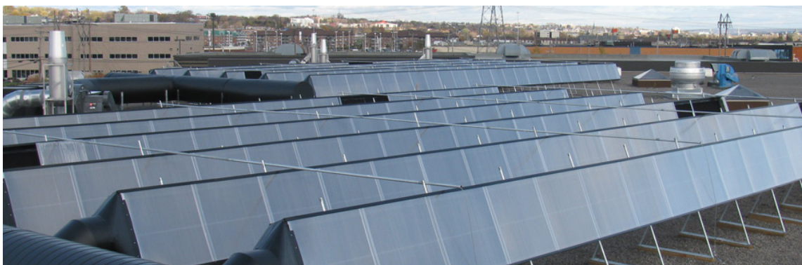
Figure 3. Part of the 144 solar collectors on the flat roof of Quebec City public transportation company bus headquarter. Each collector rapidly heats air and generates a 2.5-kW capacity on optimum solar days. (Reproduced from Ref. [18], with kind permission).
