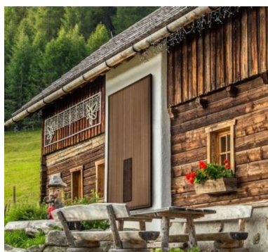
Figure 2. A glazed solar collector colored in brown for architectural integration. The panel uses a TISS nanocoating to reach high temperatures, regardless of the color. [Reproduced from solar-air.eu, with kind permission].
