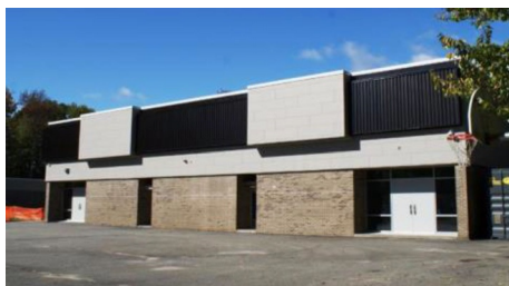
Figure 3. New York's Bedford school gymnasium after renovation to incorporate solar air collectors [Photo courtesy of Ksq Design].
