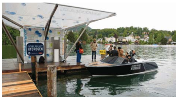
Fig. 8 The Clean Power Station makes use of a 250 m 2 flat roof equipped with PV modules whose electric power output feeds an electrolyzer splitting water molecules. (Image courtesy of Fronius).
