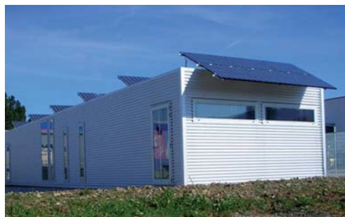
Fig. 10 The HydroLAB is completely off-grid since photovoltaic solar panels provide electricity and solar thermal vacuum tube panels provide heat for room heating and feed a solar cooling machine (5 kW, the smallest in Italy) in order to get air conditioning at zero emission in summer. (Photo courtesy of La Fabbrica del Sole).
