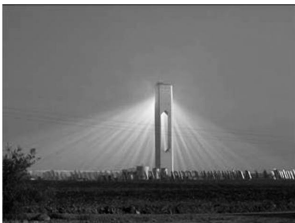
Figure 1. The Solucar 11 MW solar thermal plant outside Seville, Spain, produces enough electricity to power 6000 homes. Concentrated solar power is the large-scale technology capable to satisfy massive electricity demand (photo courtesy of the BBC).
